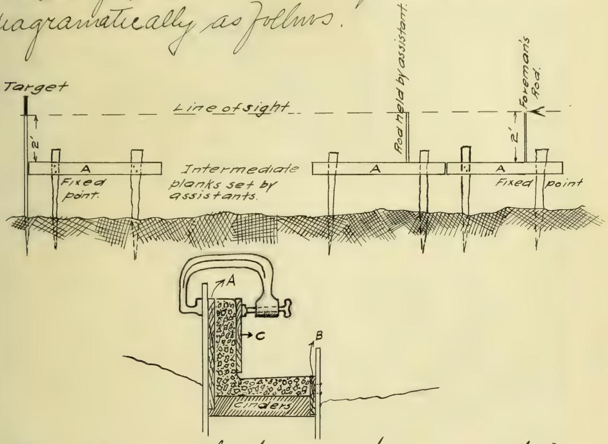
After placing the backing boards (A) the front boards (B) are placed at a distance from A equal to the curb thickness plus the width of the gutter flag. These too are held in place by stakes, and are so graded that the fall in the gutter toward the inlets is as prescribed in the profile. Their elevation is fixed by measuring down from the backing boards, already fixed.
